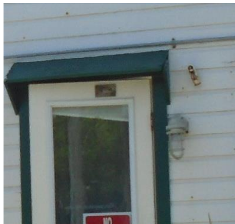
Light fixture with exposed bulb does not conform to the Town Code.
