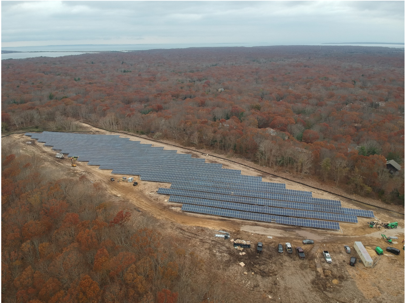
Work in progress, November 19, 2018
